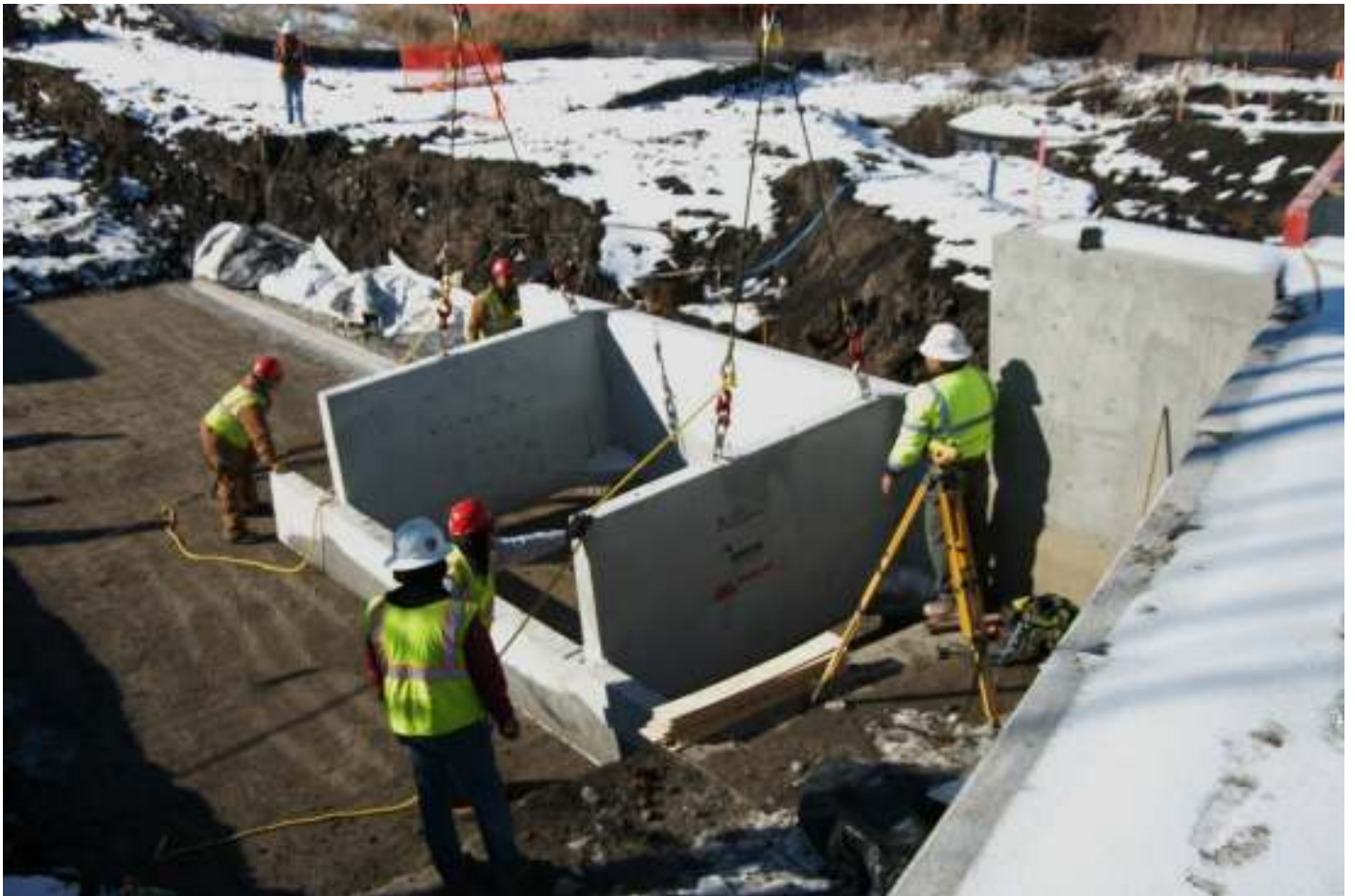
Designed for easy and fast construction using big equipment for best filling and compaction.
