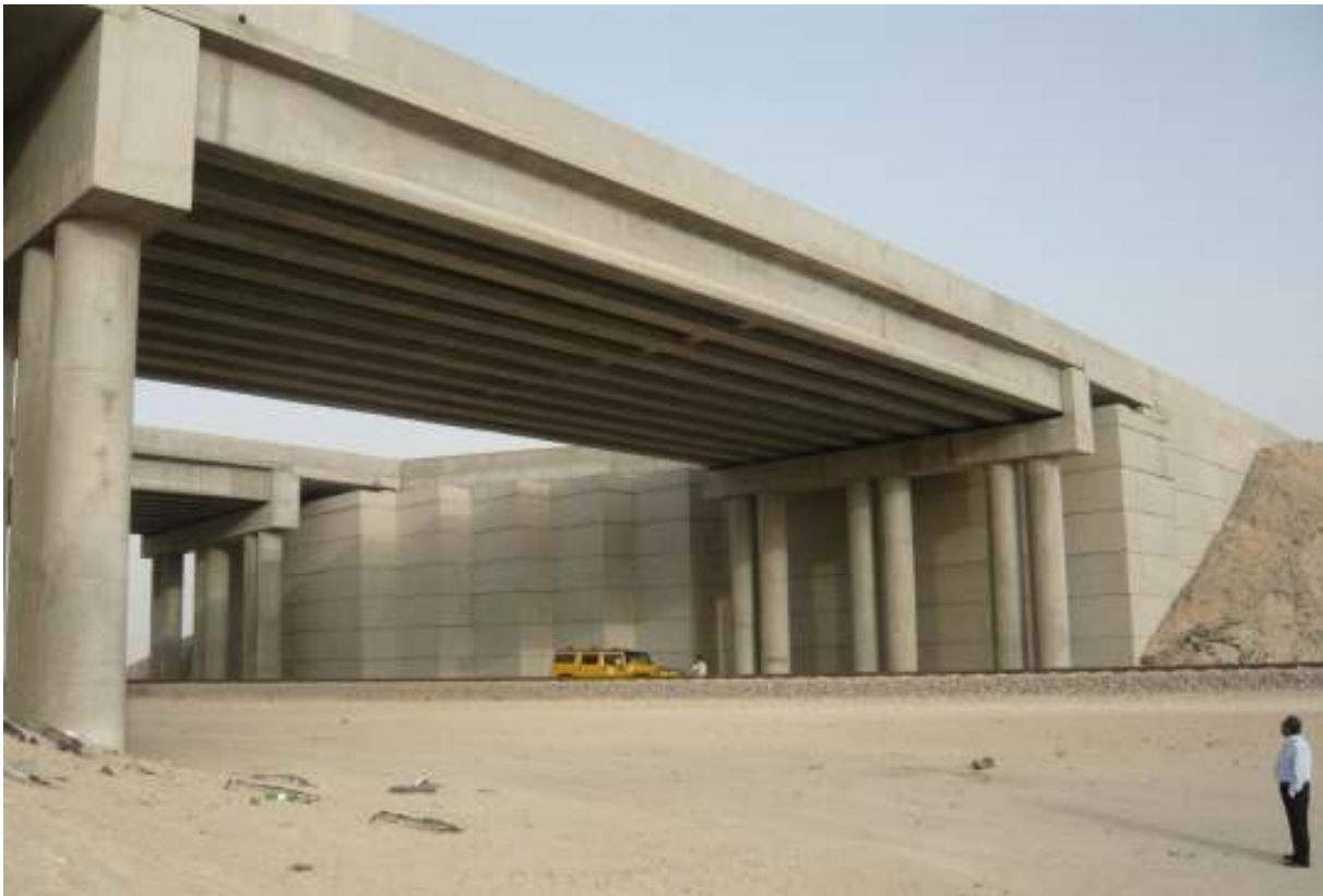
Rail road crossing for six lane highway in Saudi Arabia - Special Corner Design and Completion
